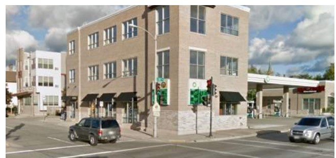
Figure 3.170-B. Example of Fuel Station
