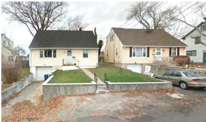
Figure 3.100-G. Basement Garage on House B Building
