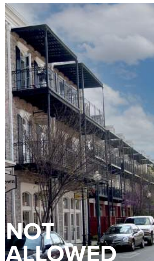
Balconies: Covers More than Allowed Facade Area
