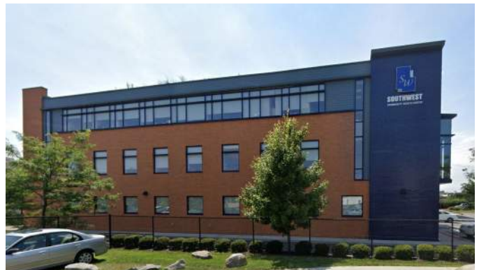
Figure 3.50-A. Examples of General Building Type
